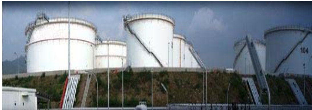
Benzene storage tanks
