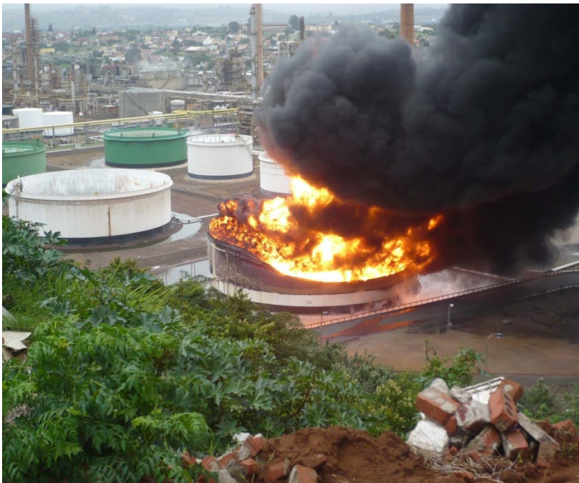
November 2007: Storage tank fire at Engen refinery. Fire burned for five days
